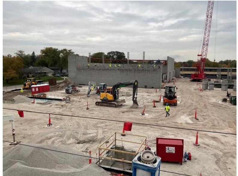
Last gym masonry wall topping out.
