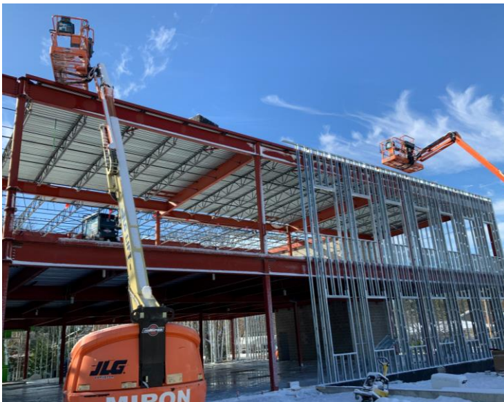
Steel roof decking installed for second floor classrooms.
