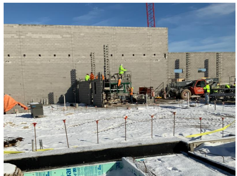
Music masonry wall construction.
