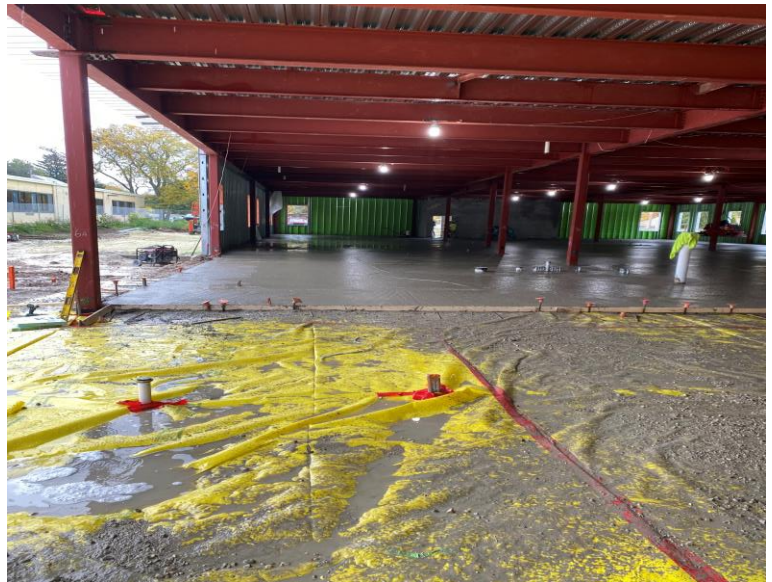
First floor concrete slab being installed.
