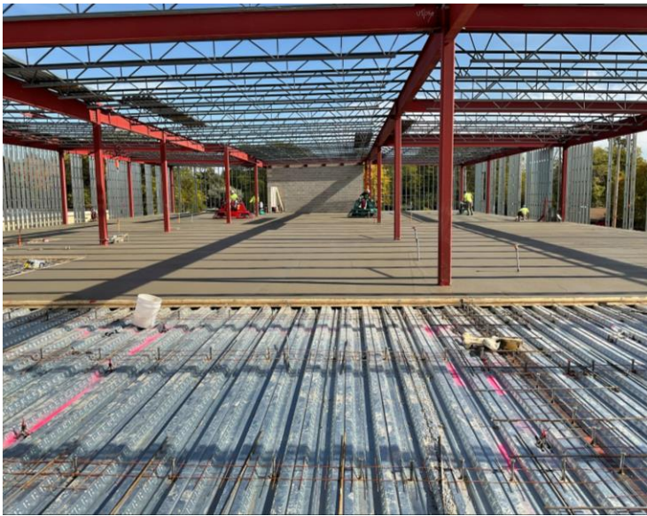
Concrete deck was poured for the second floor classrooms.
